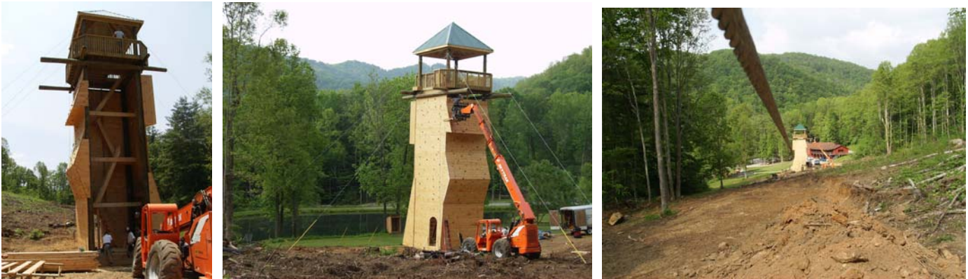
New King Climbing Tower Under Construction
