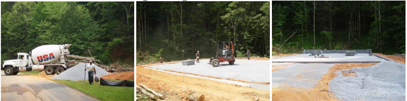
Pavilion Pad in Progress
